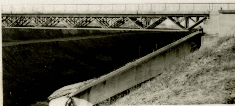
Co. "B" BUILT A DOUBLE-DOUBLE BAILEY OVER THIS RAP. LOCATED NEAR THE HUGE OPEN SURFACE ALINE ON THE ROAD BETWEEN WEISCHWILLER AND DÜREN.
